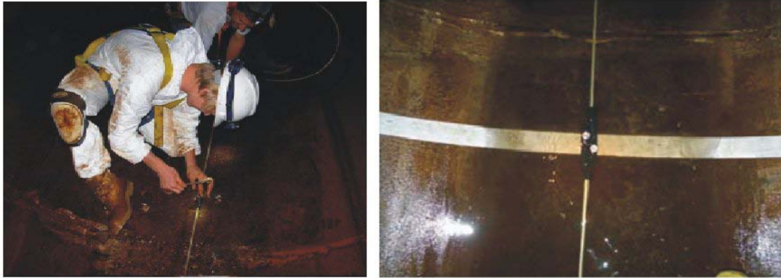
Figure 3-29. (Left) Installation of Fiber Optic Sensor in a Dewatered Pipeline. (Right) Fiber Optic Sensor Installed on a Stainless Steel Hoop with a Strain Relief Device (Reprinted with permission from Pure Technologies)
