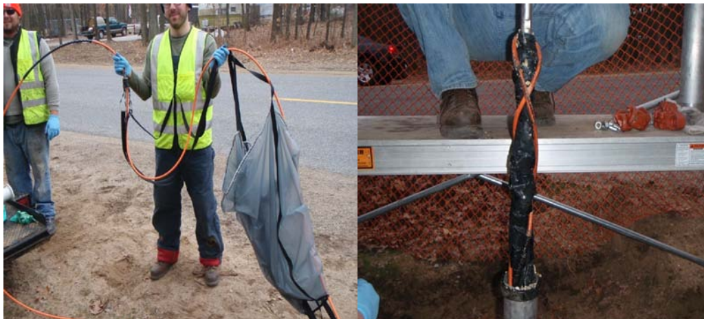
Figure 3-30. (Left) Installation Parachute Used to Install an AFO Cable in an in-Service Pipeline and (Right) Parachute Caught and Extracted at Two Miles Downstream from Insertion Point (Reprinted with permission from Pure Technologies)
