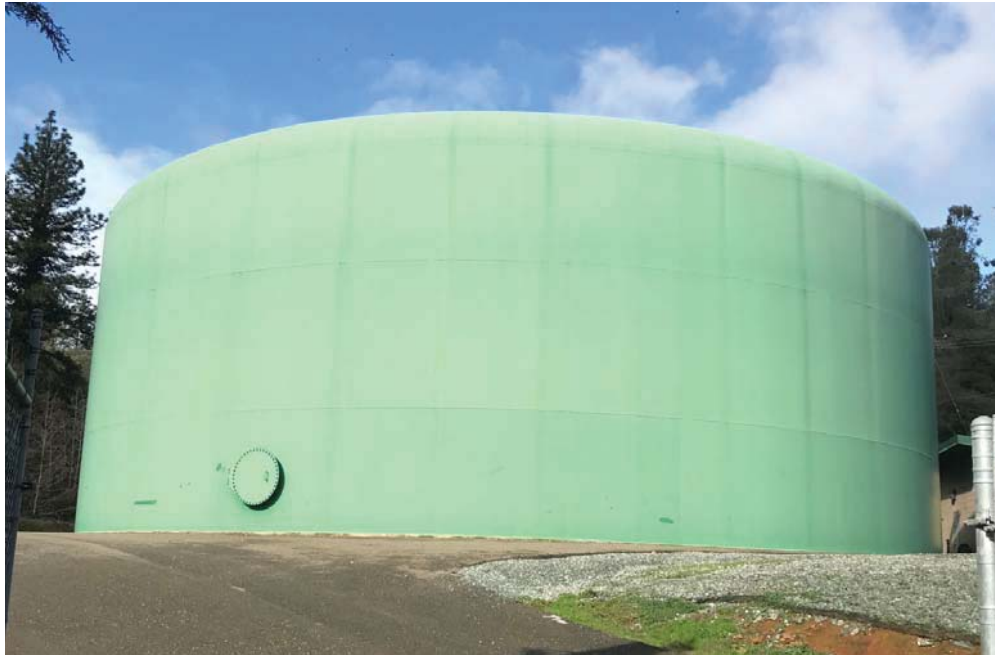
Photo #7) View of similar tank from 80 feet away.
