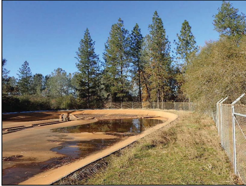
View of existing reservoir. Photo date 12-7-17.
