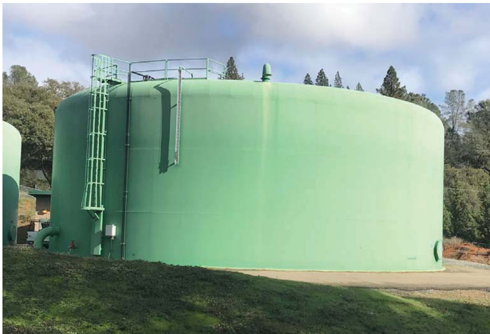
Photo #8) View of similar tank from 125 feet away.
